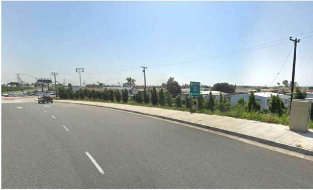
VIEW ON 405 FWY OFF-RAMP LOOKING SOUTHEAST 5
